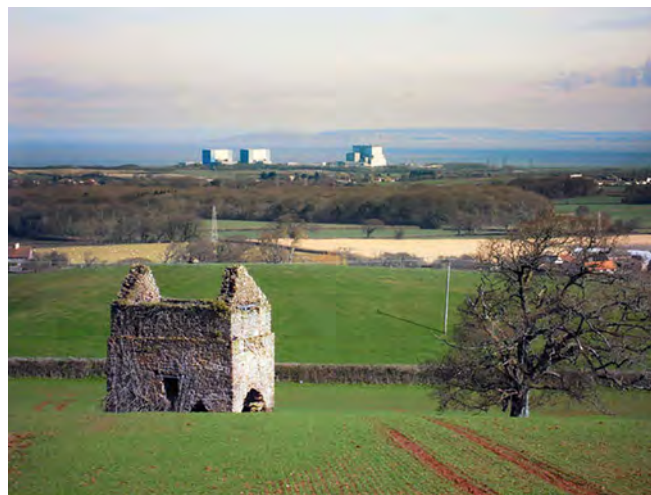
Glebe engine house; Hinkley Point power station is seen in the distance. Photo Nick Chipchase
